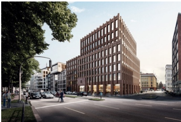
The Tichelhaus property with its elegant brick façade
